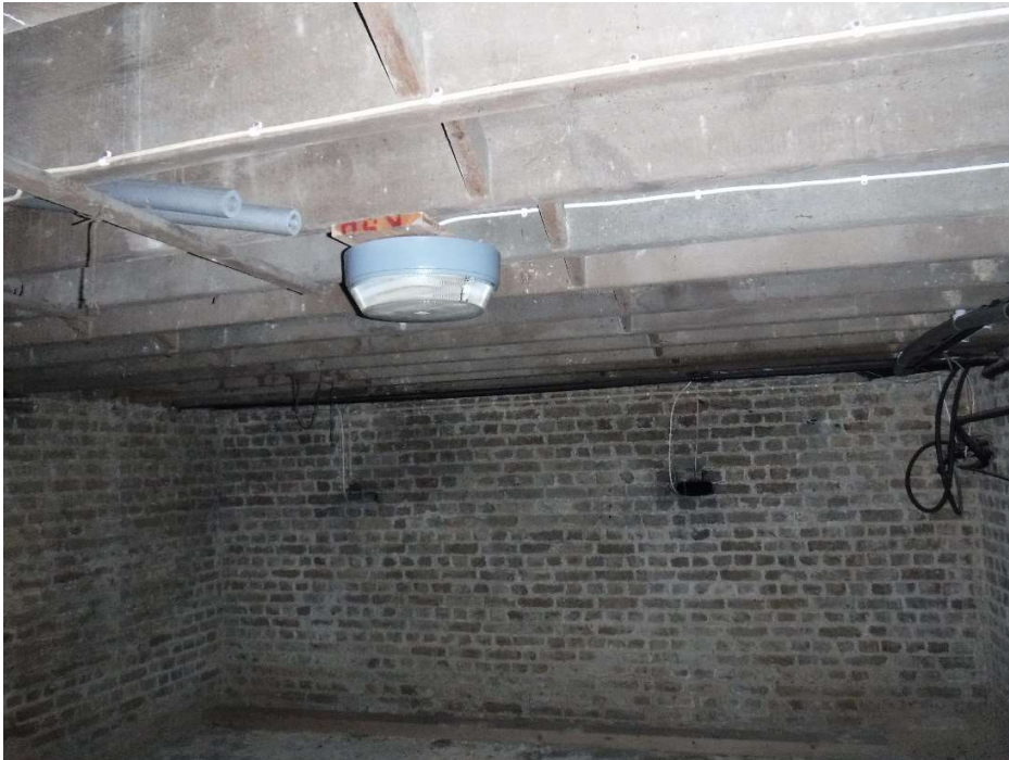
Photograph 004 – General view of Basement Area B
