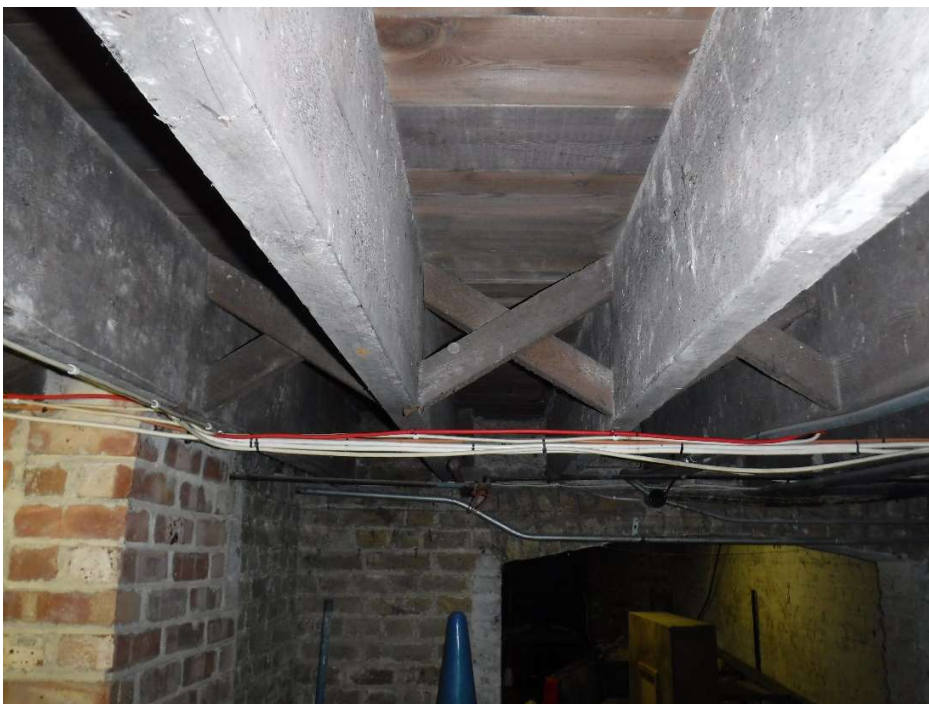
Photograph 002 – View of soffit with beams and cross bracing
