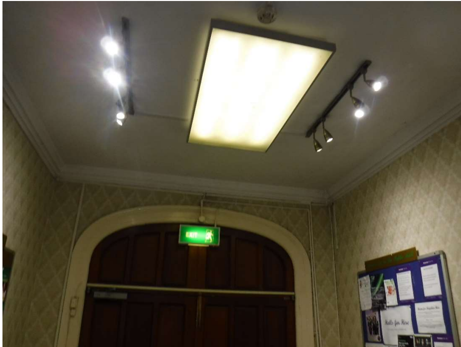
Photograph 012 – General view of “lobby” Area G
