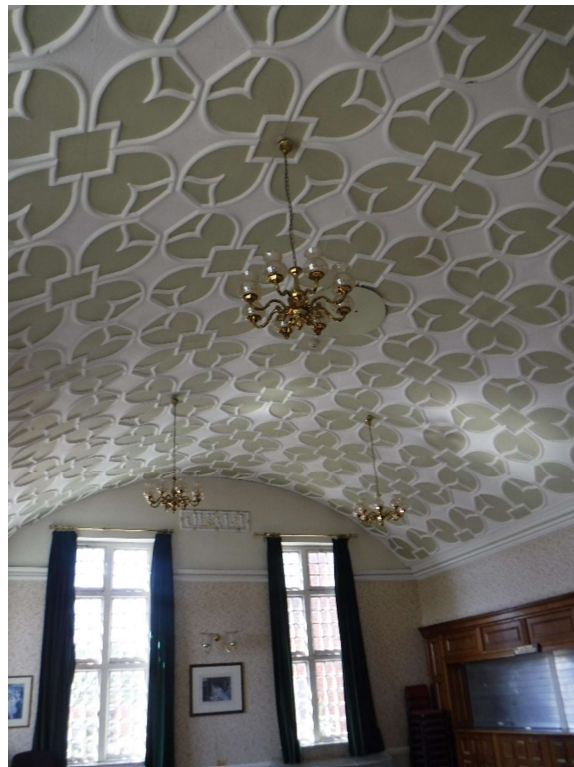
Photograph 038 – General view of Area V Soffit
