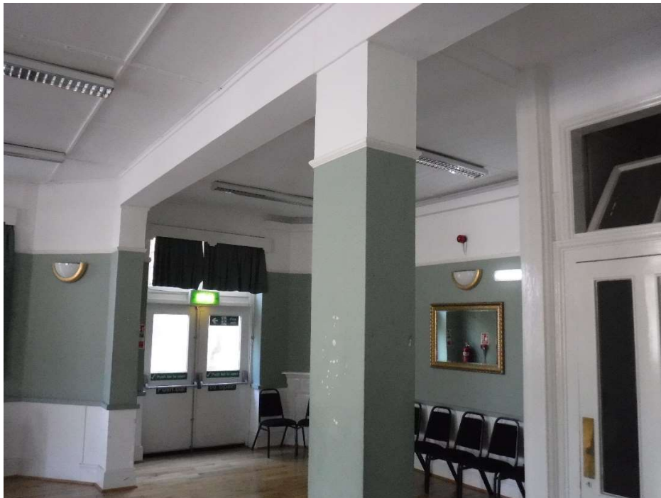
Photograph 010 – General view of column line in first floor Area F
