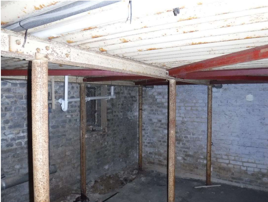
Photograph 008 – General view of construction in Area D
