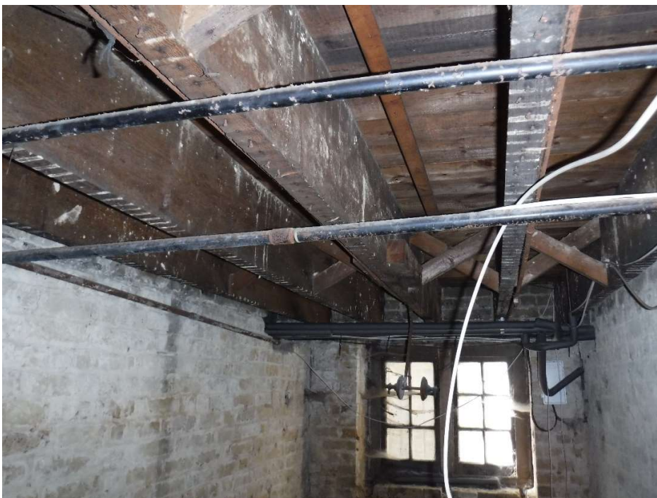
Photograph 009 – Timber construction of floor in Area D
