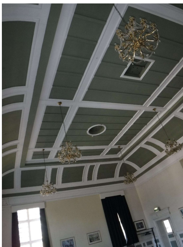
Photograph 026 – General view of ceiling within area P
