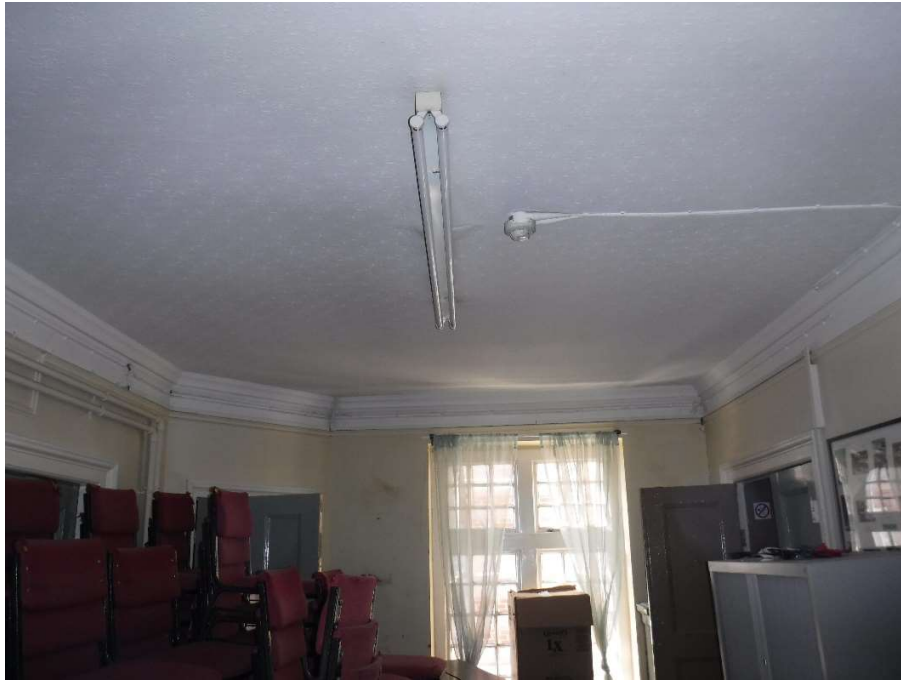
Photograph 035 – General view of Area T
