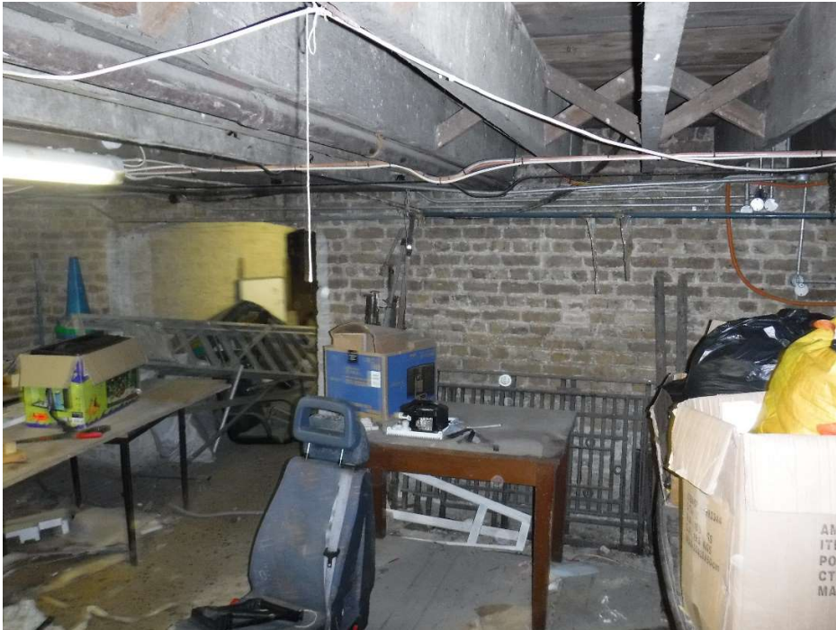
Photograph 001 – General view of Basement area A
