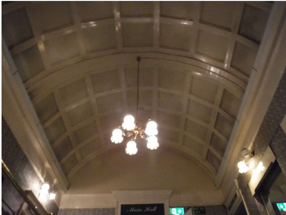
Photograph 034 – General view of Area S ceiling
