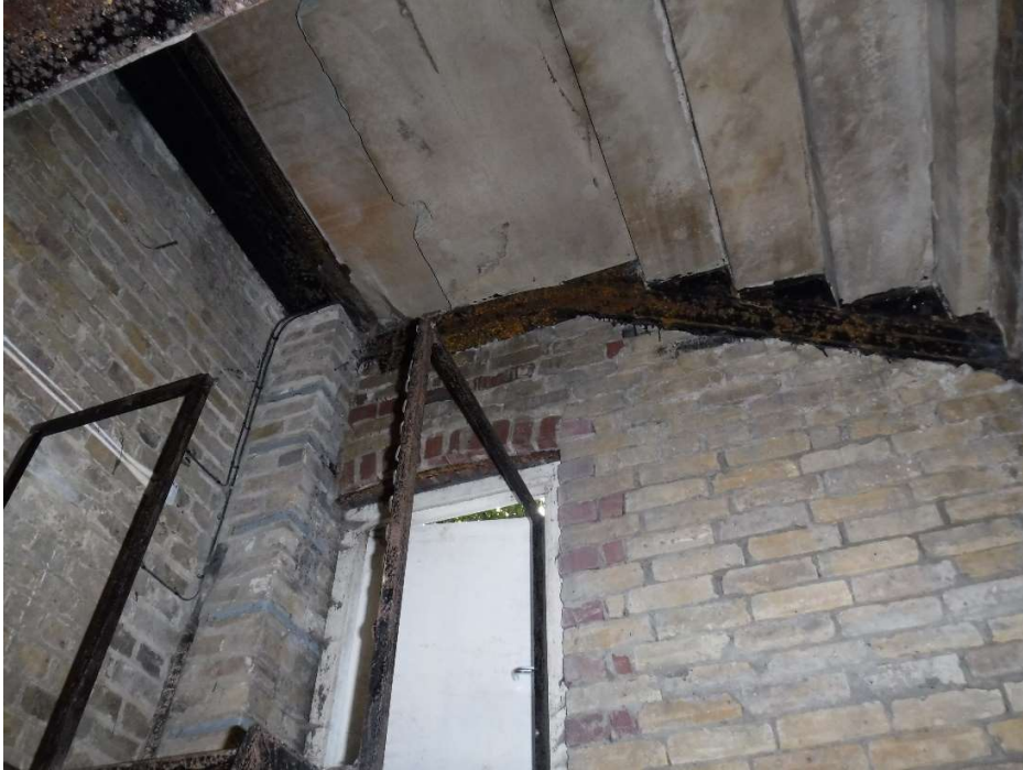
Photograph 006 – General view to underside of stairs within Area B
