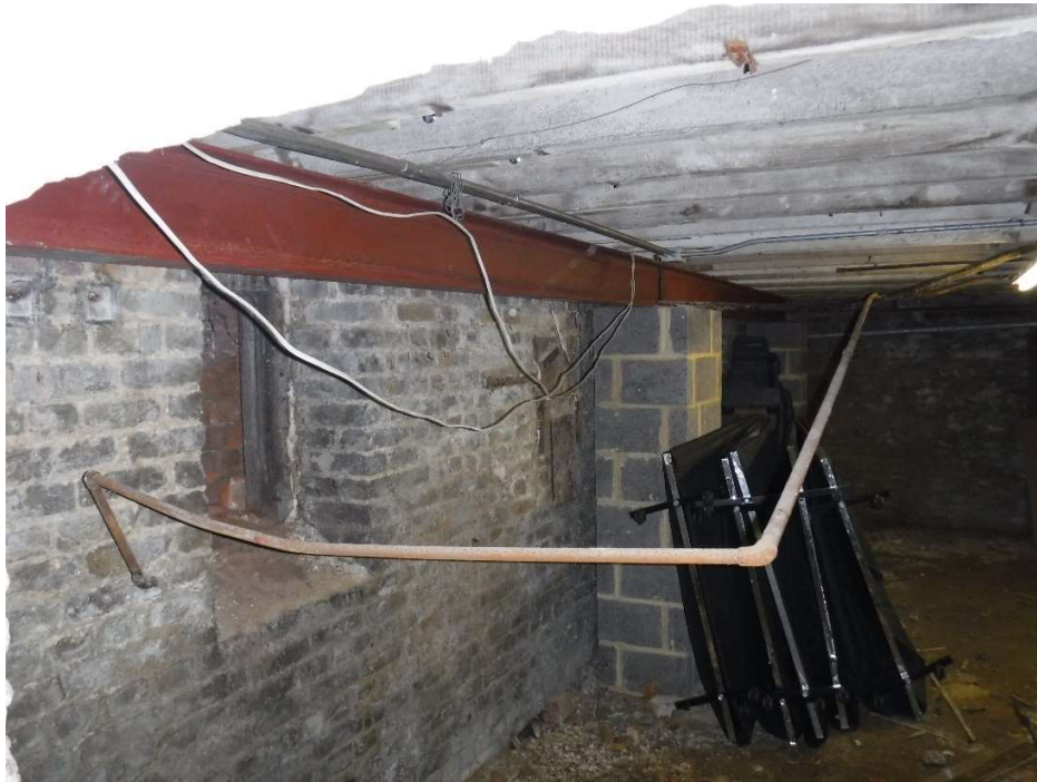
Photograph 003 – Steel I Beam situated on masonry piers
