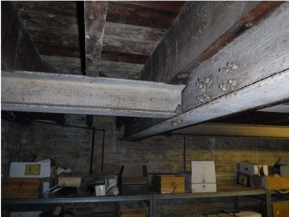
Photograph 007 – General view of floor construction and beams beneath in Area C
