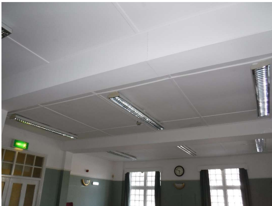
Photograph 011 – General view of beams and ceiling in Area F
